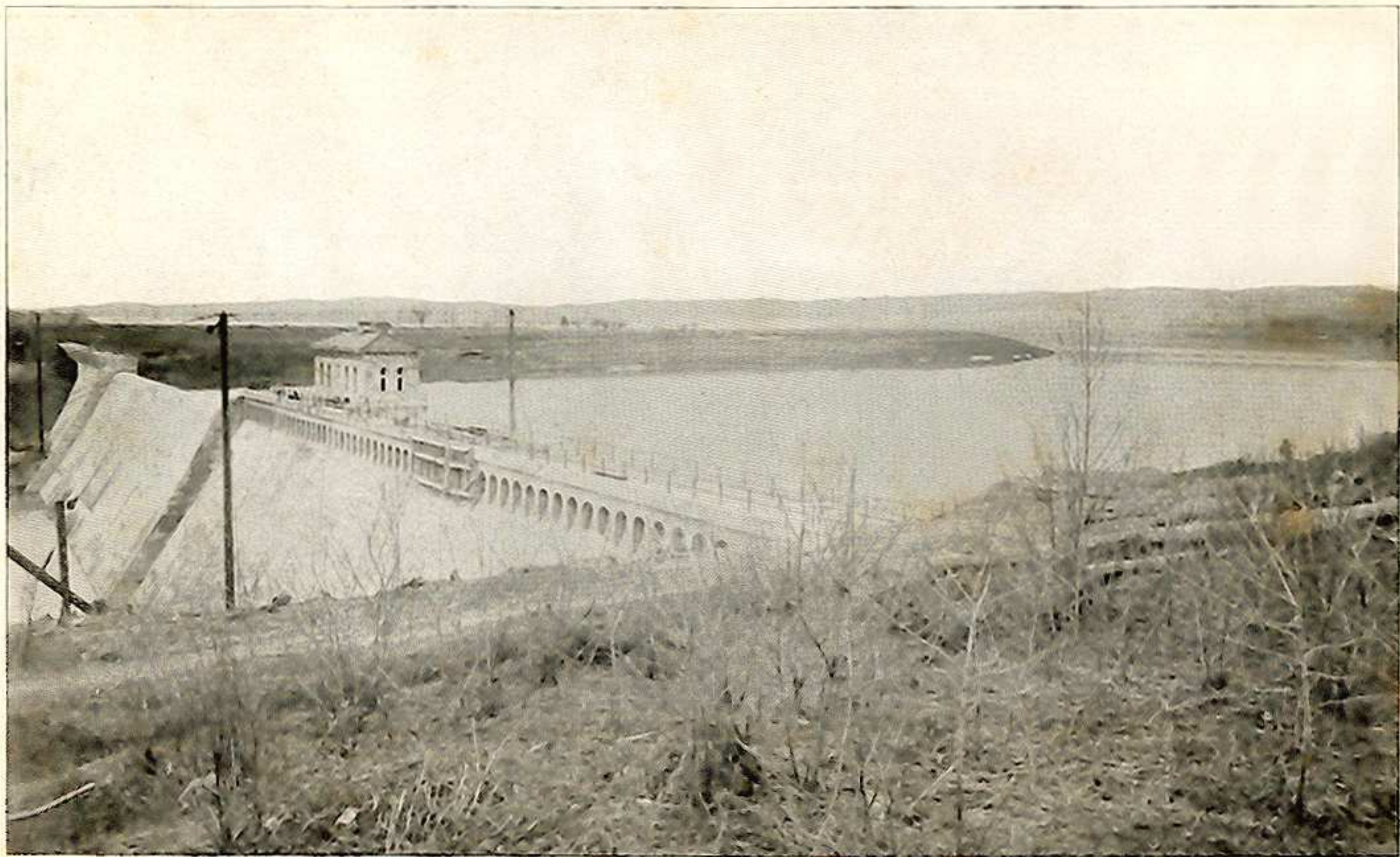
View of the completed dam at Delta reservoir, showing the partially filled reservoir. The dam, which is 1,100 feet long and stands 100 feet high above the lowest foundation, forms a lake two miles across at its greatest width and four miles long. This is one of the two large reservoirs added to the State water storage system for supplying the canal.
