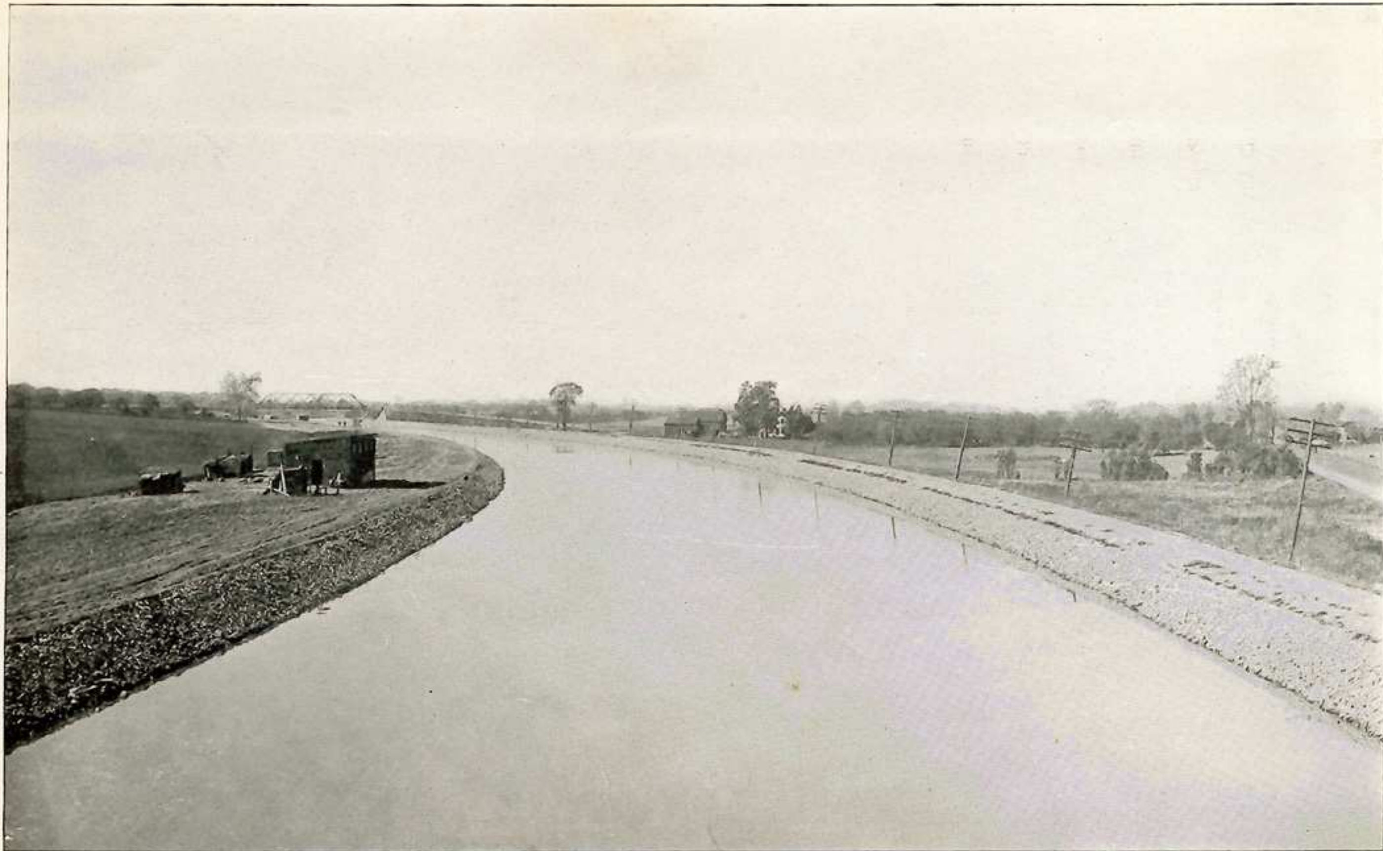
Completed channel, typical of the Rochester-Lockport level, where in general the alignments of the Barge canal and the present canal are identical.
